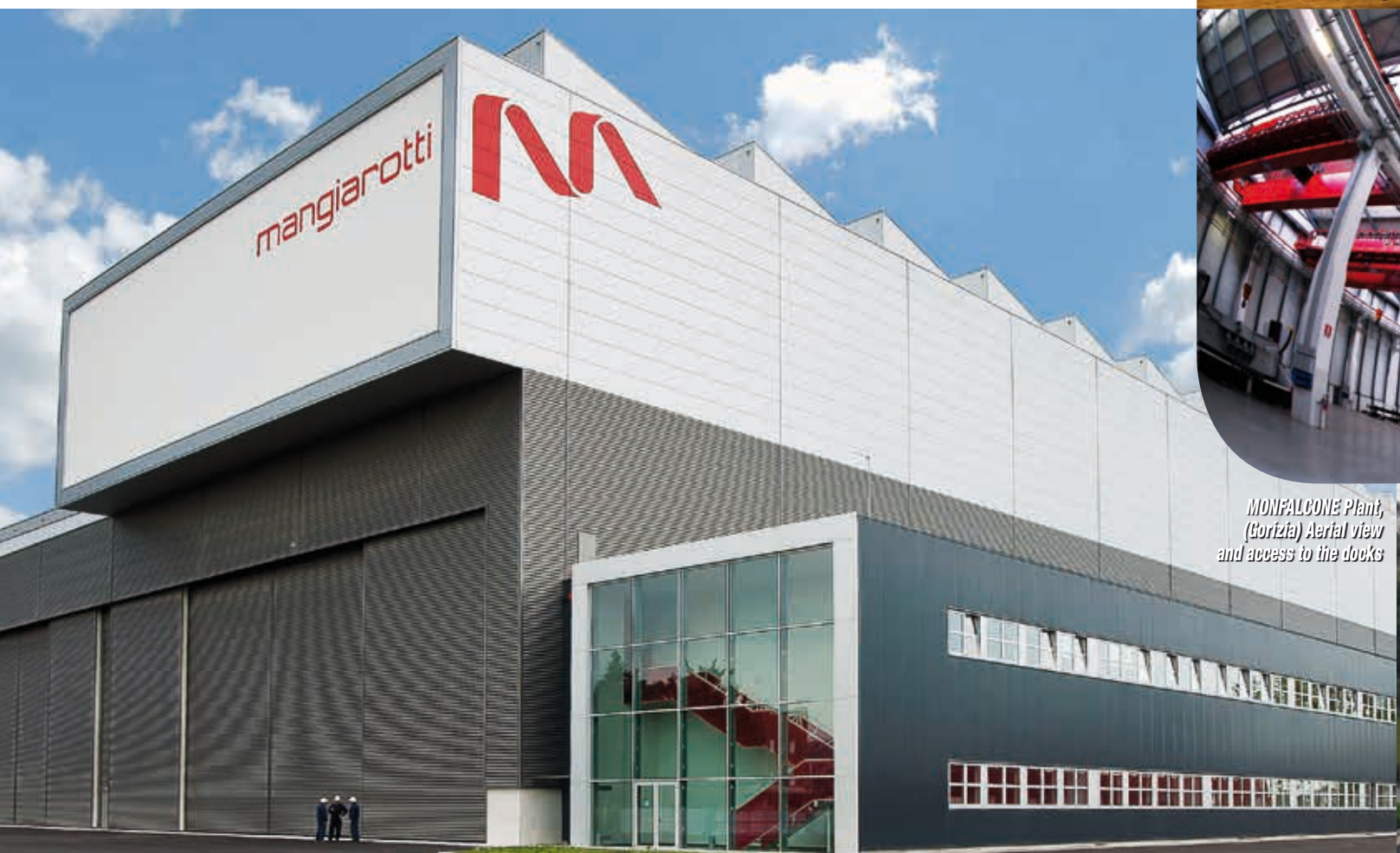
MONFALCONE Plant, (Gorizia) North view
